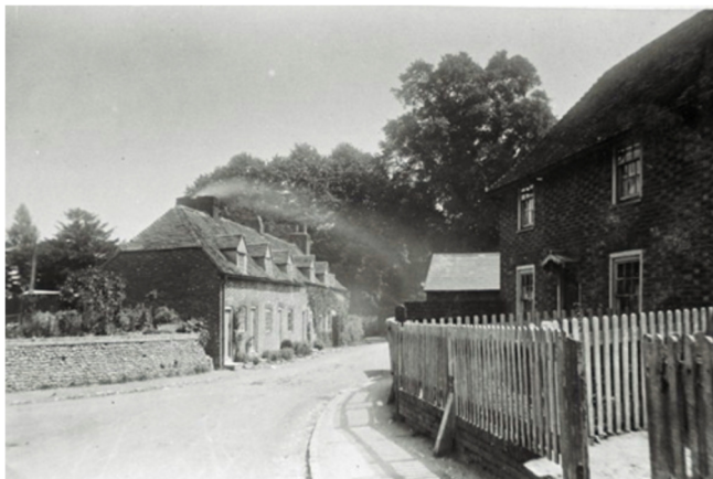
(This picture shows the original Ivy Cottages, looking in the direction of Bucks Cross from the village centre.)
